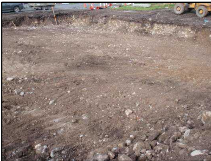
Plate No. 7 Upper level reduced to formation level, from S.
