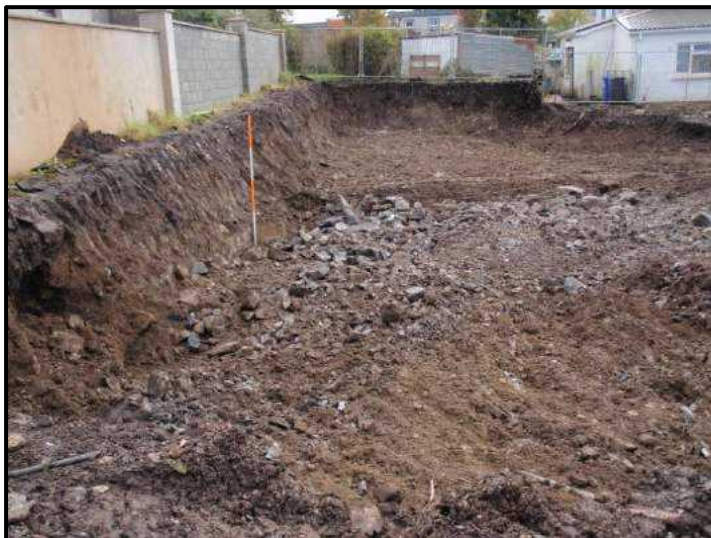
Plate No. 9 Looking SE across Site B reduced to formation level, showing bedrock (C9).
