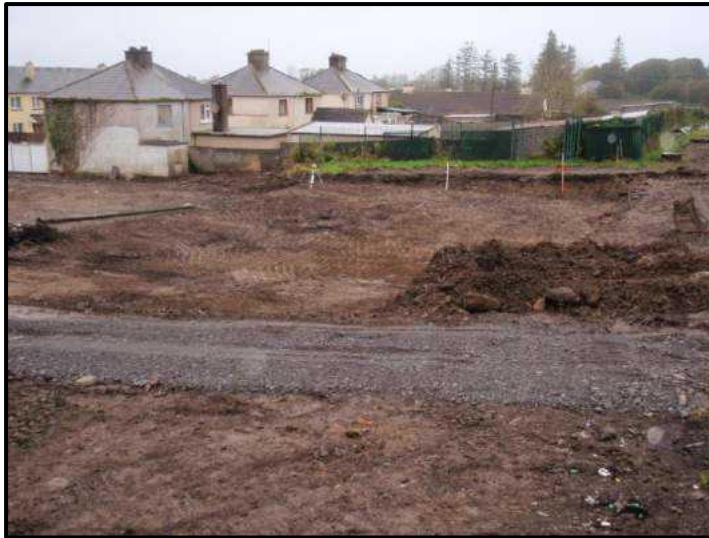
Plate No. 6 Central level reduced to formation level, from E.
