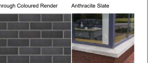
Dark Brick & Light Colour Mortar Precast Concrete Cills
