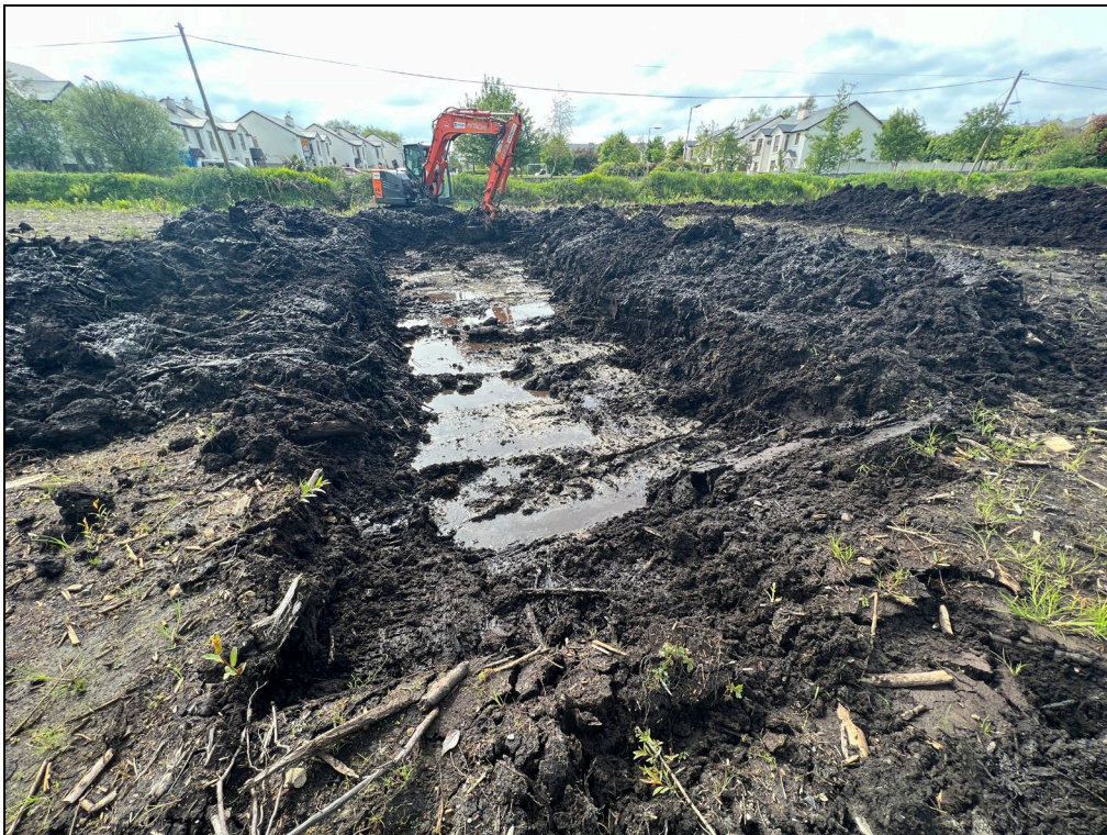
Plate 22: West facing view of Test Trench 12.
