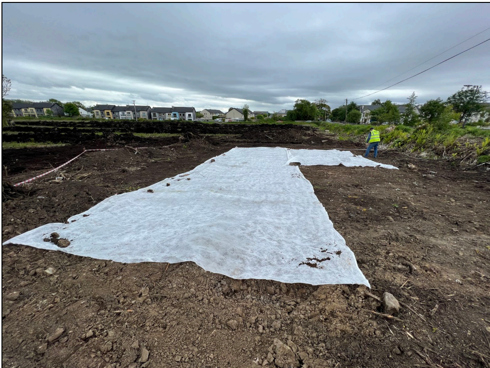
Plate 16: South facing view of the burnt mound after covering with terram.
