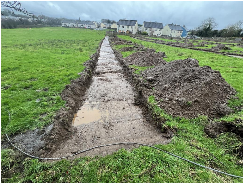
Plate 9: South facing view of Test Trench 6.
