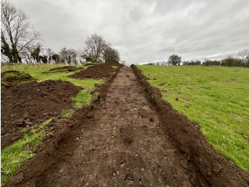
Plate 4: North facing view of Test Trench 1.
