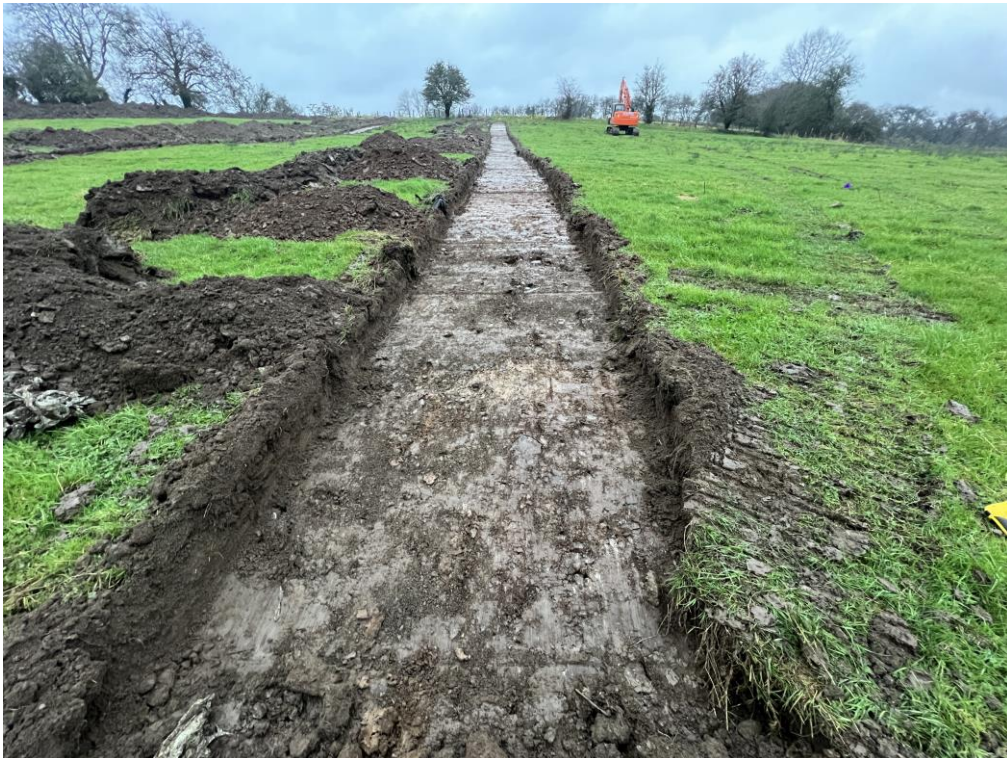
Plate 7: North facing view of Test Trench 4.
