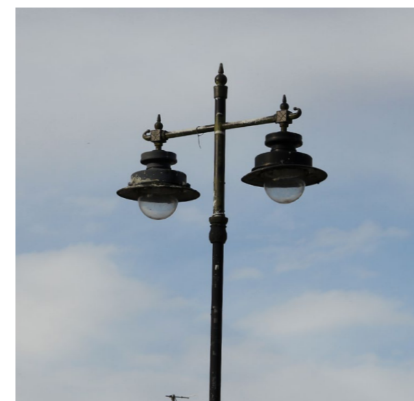
Refurbishment of existing light columns
