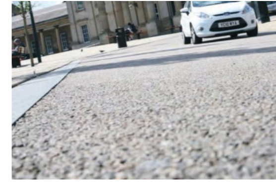
Light grey coloured asphalt to parking bays
