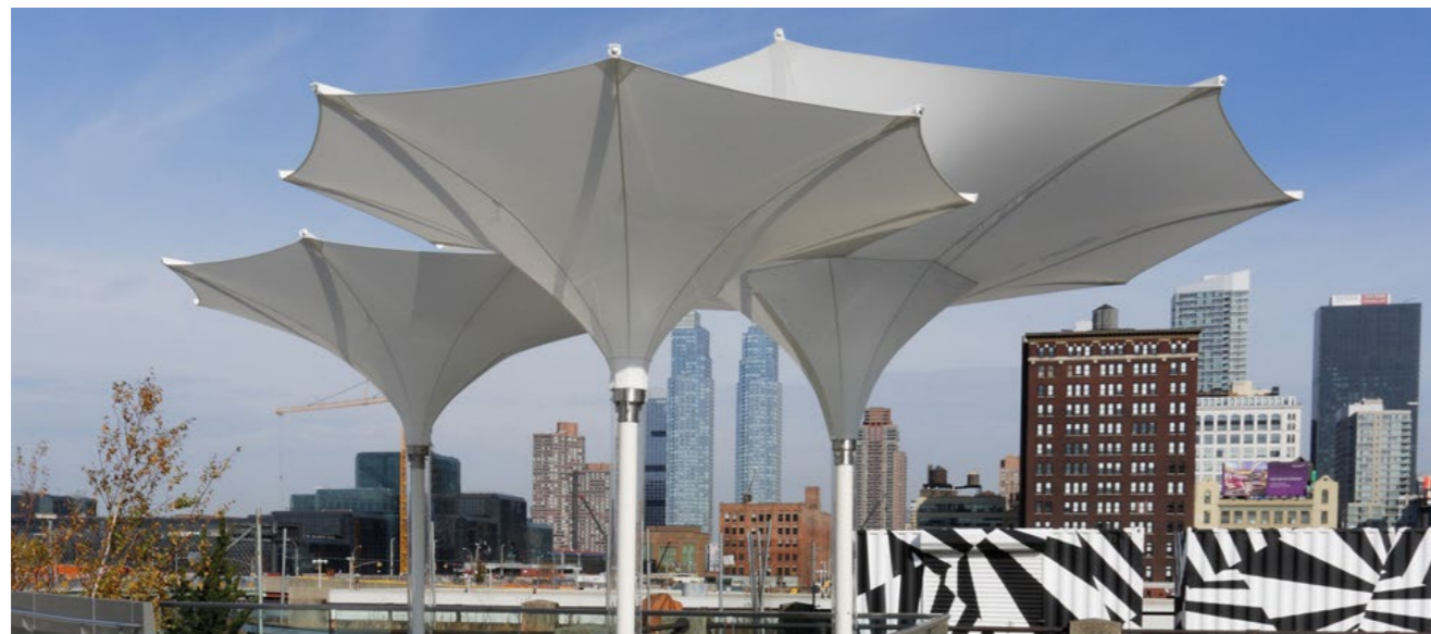
Proposed umbrella forest shelter, or similar shelter. Approximate height 4 - 4.5m to enable clearance for vans beneath structure on market days
