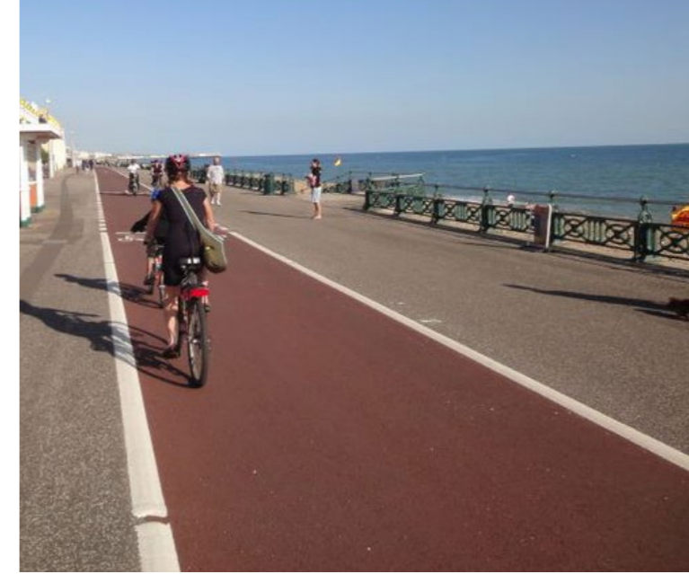
Example of coloured asphalt used to demarcate cycleways
