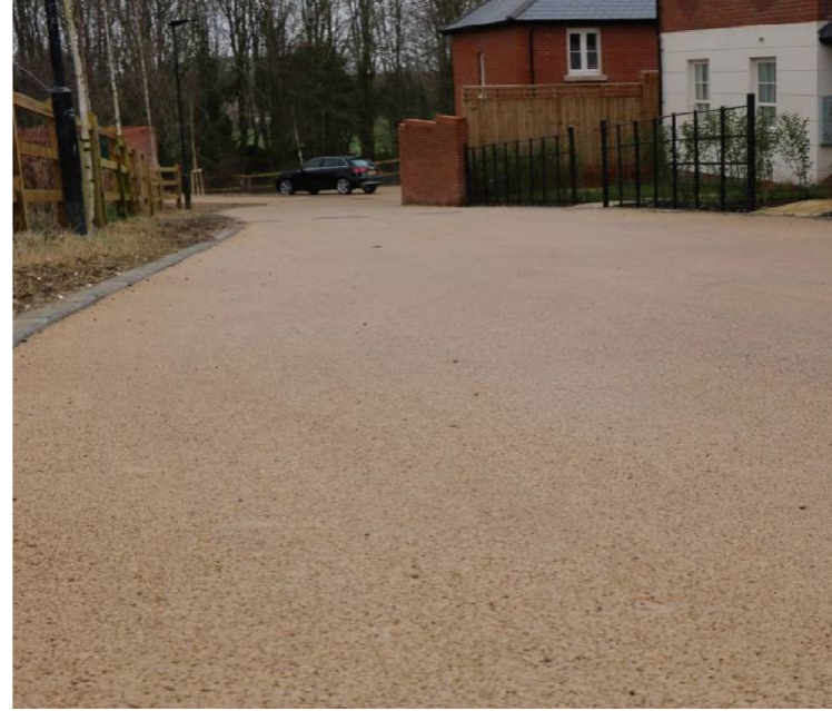
Example of coloured asphalt
