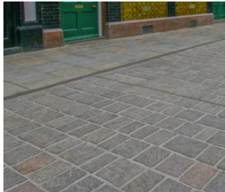
Example of natural stone paving with a traditional finish and colour variation
