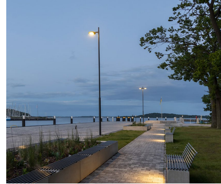
Example lighting column
