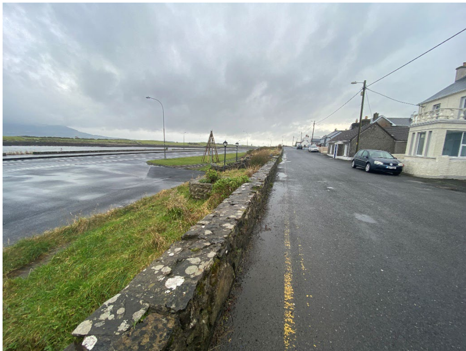
Plate 6 West facing view of the carpark and old road outside The Driftwood
