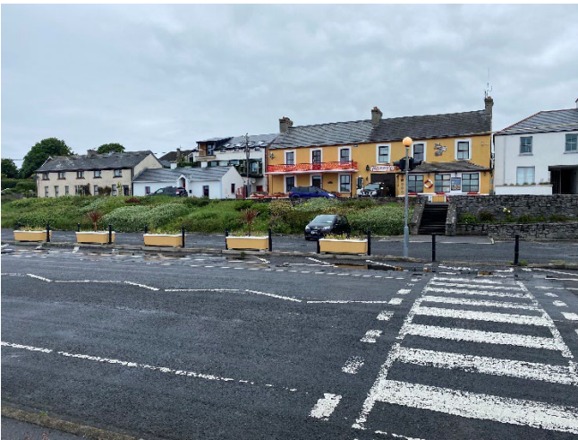
Figure A7: Location of proposed parking resurfacing, raised table crossing and planting outside Harry's
