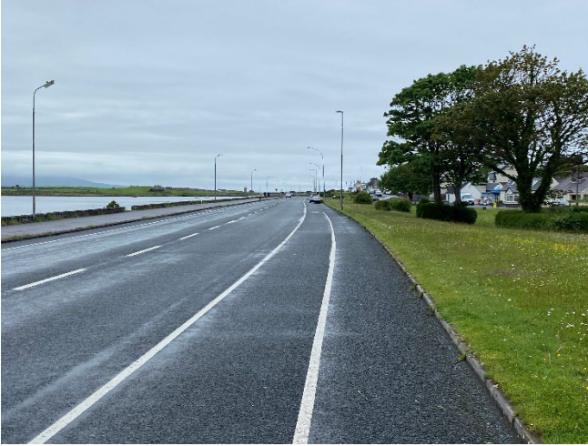
Figure A5: Existing hardstanding section along New Road to be demarcated for parking
