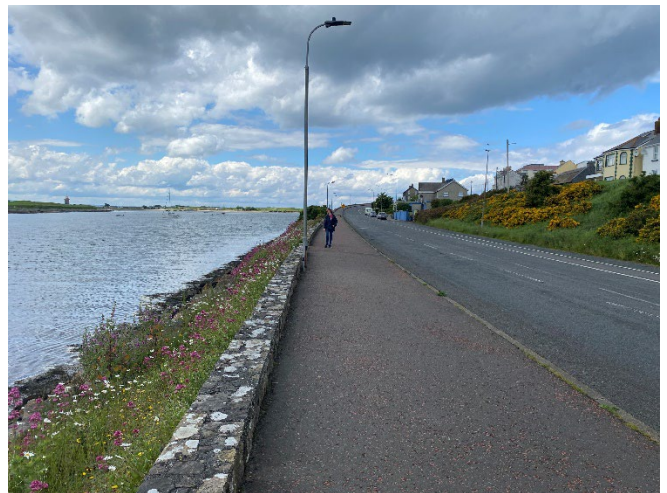
Figure A4: Existing footway surfacing retained to southern boundary wall to harbour
