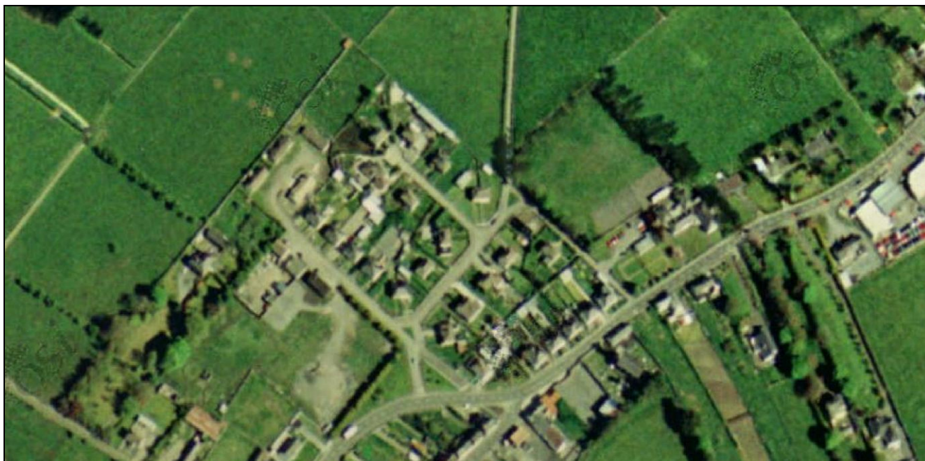
Figure 1: historic aerial view of the development at Connolly Park. Circa 2000 Courtesy of OSI. Licence number 2020/30/CCMA/ Sligo County Council
