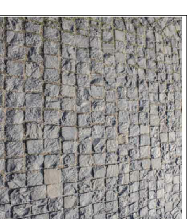
2 GRANITE Limestone CUBES - REGULAR LAYOUT OR SPAYED CIRCULAR LAYOUT - TO BE DECIDED AT DETAILED DESIGN STAGE
