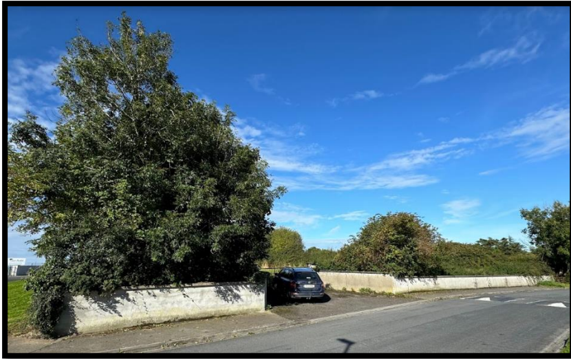
Block wall enclosing the old reservoir.
