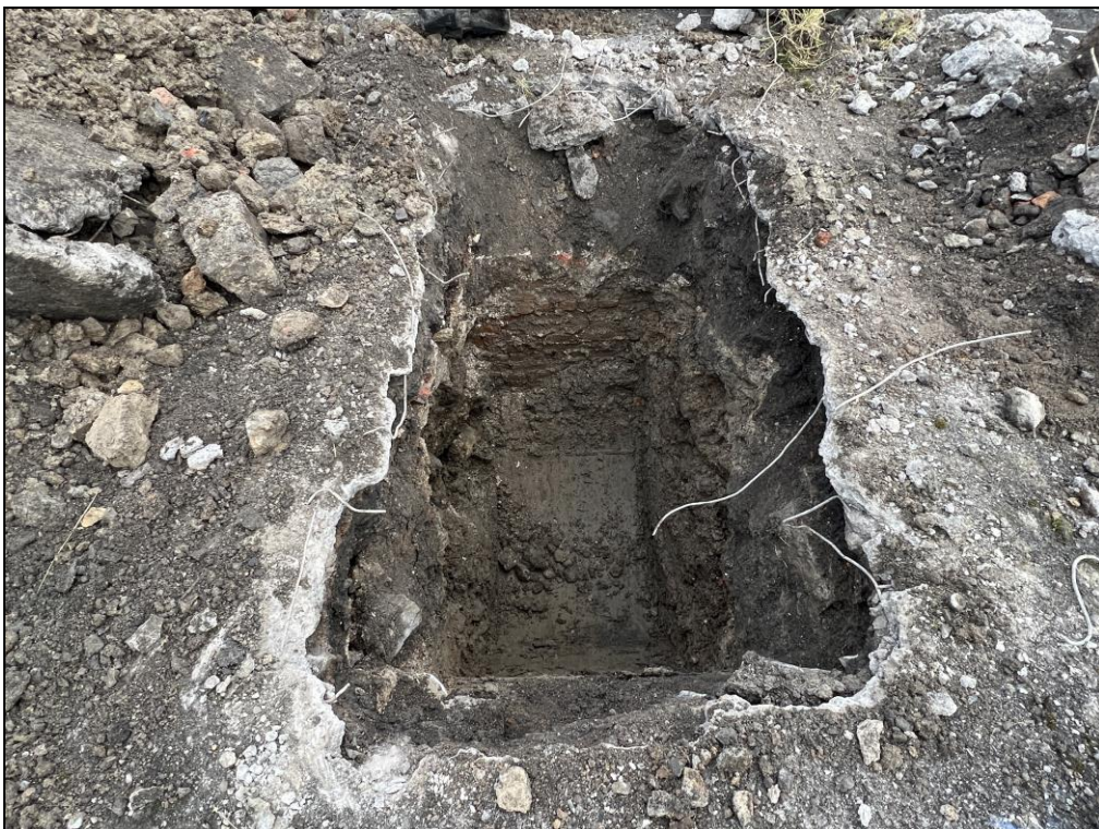
Plate 12: East facing view of Trial Trench 5 showing the brick wall.
